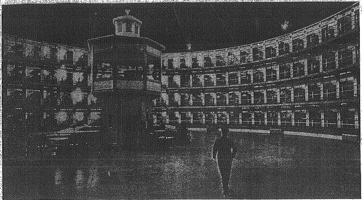
Stateville prison: In 1925, the circular glassed-in cell blocks were the last word in penitentiaries
